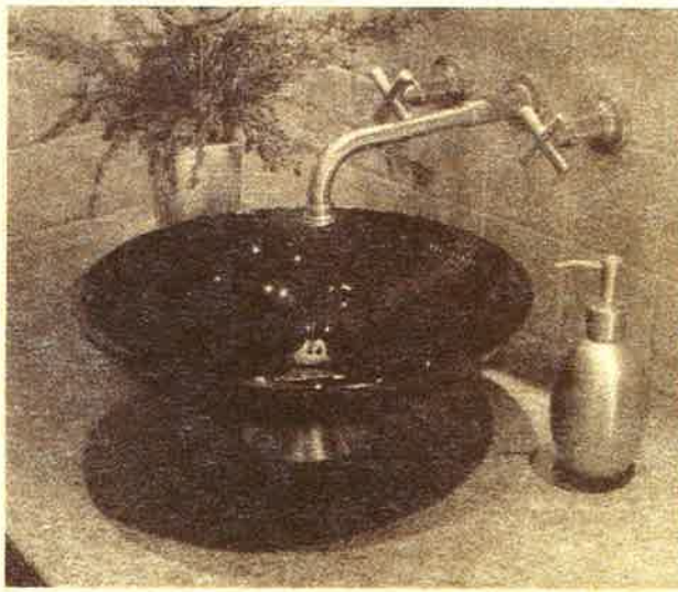
Above-counter vessels have become very fashionable in recent years as an alternative to standard bathroom sinks. John Ambrose of Sun Remodeling combined this vitreous glass bowl, made by Hectarus of Canada, with a wall-mounted faucet finished in brushed nickel to make quite a fashion statement in this bathroom remodel. Photo courtesy of Sun Remodeling.
